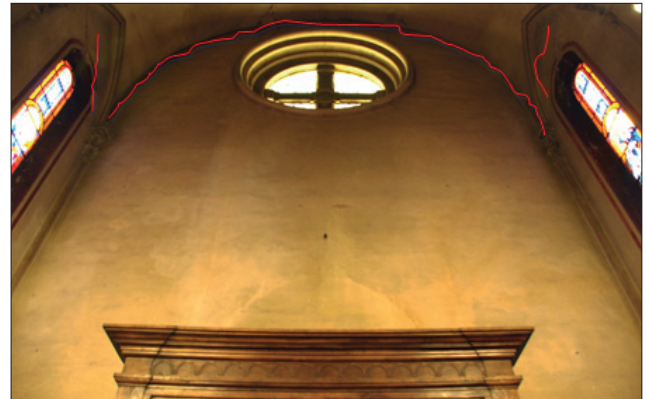
FIGURE 17 Façade overturning mechanism (M1), internal view
