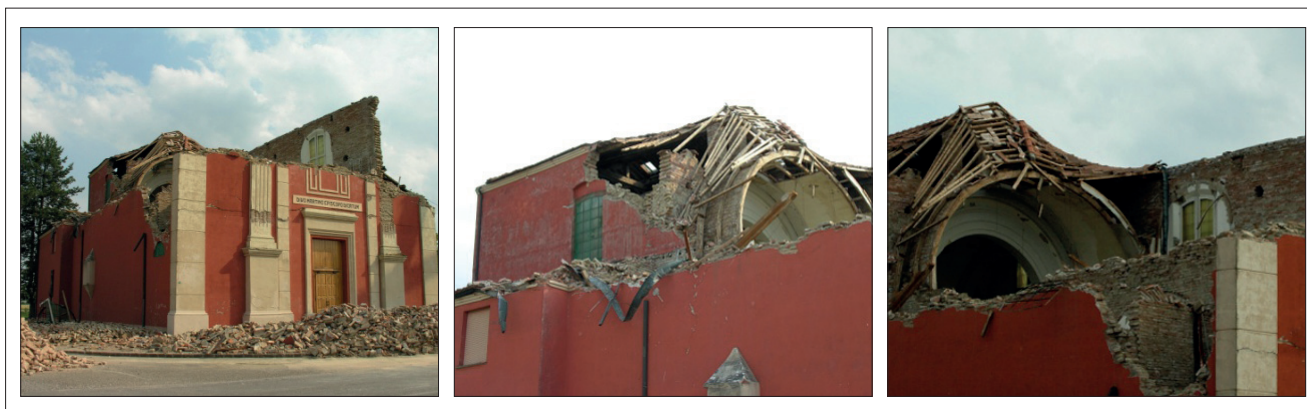
FIGURE 16 Church of S. Martino, Buonacompria, Cento (FE)
