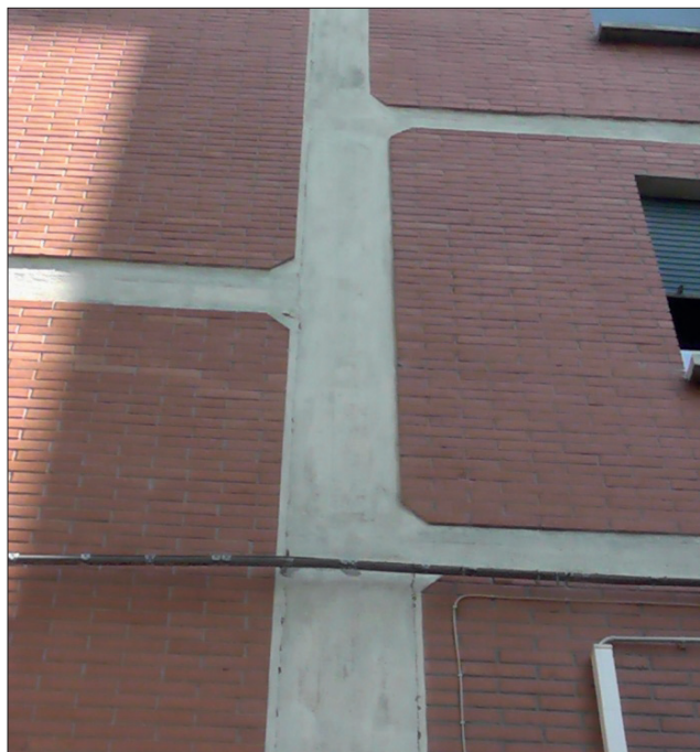
FIGURE 26 Separation between adjacent buildings
