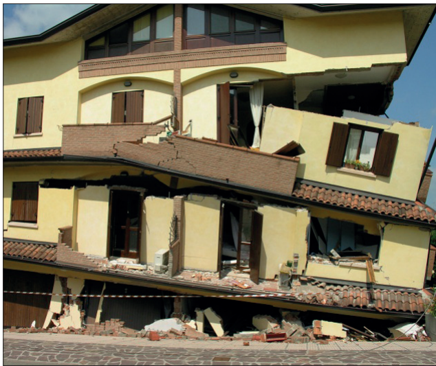
FIGURES 11-12 The soft storey has collapsed, the damage grade is 5
