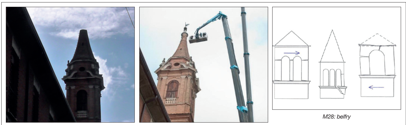
FIGURE 12 Cento (Ferrara) historic centre: the Church of San Biagio and main collapse mechanisms
