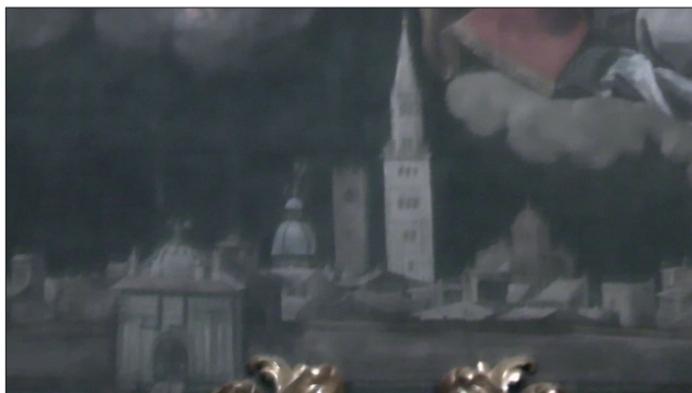
FIGURE 2 Detail of “Torre Mozza” before its demolition (on the left from the Ghirlandina Tower), from a painting located in the Modena Municipality Palace
