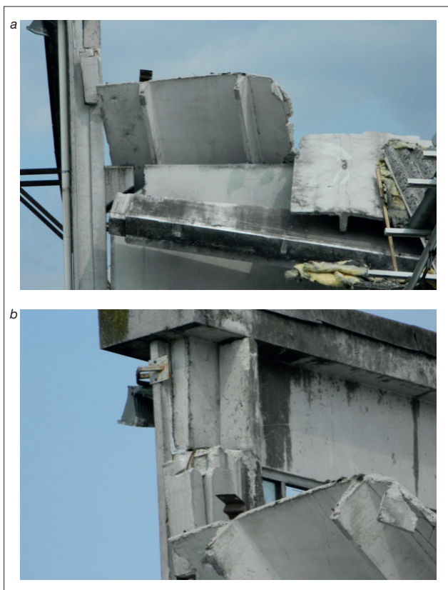
FIGURE 10 Lateral toppling of the beam Source: ENEA
