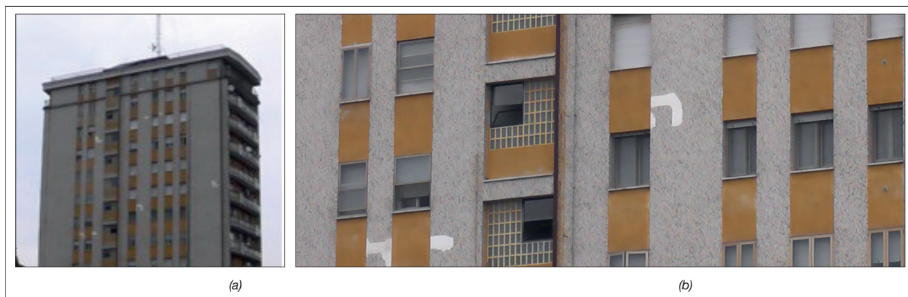
FIGURES 29 The Cento Skyscraper: a) external view; b) detail of the main façade
