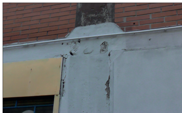
FIGURE 28 Separation between cladding and structure elements
