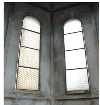
Internal iron frame of the small towers
