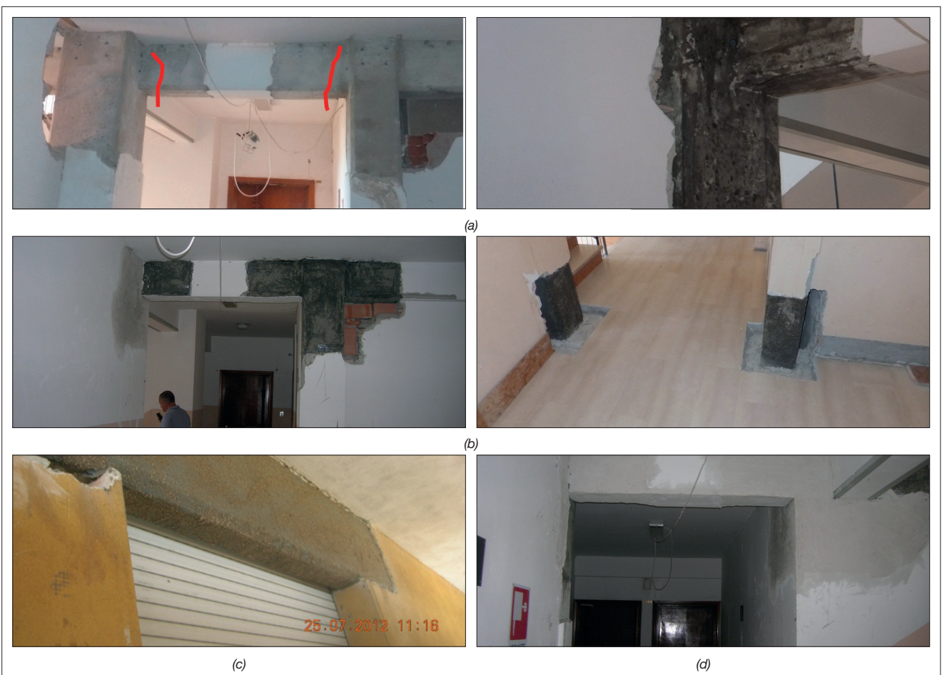
FIGURE 34 Local consolidation system: a) preparation phase; b,c) FRP application; d) plaster application
