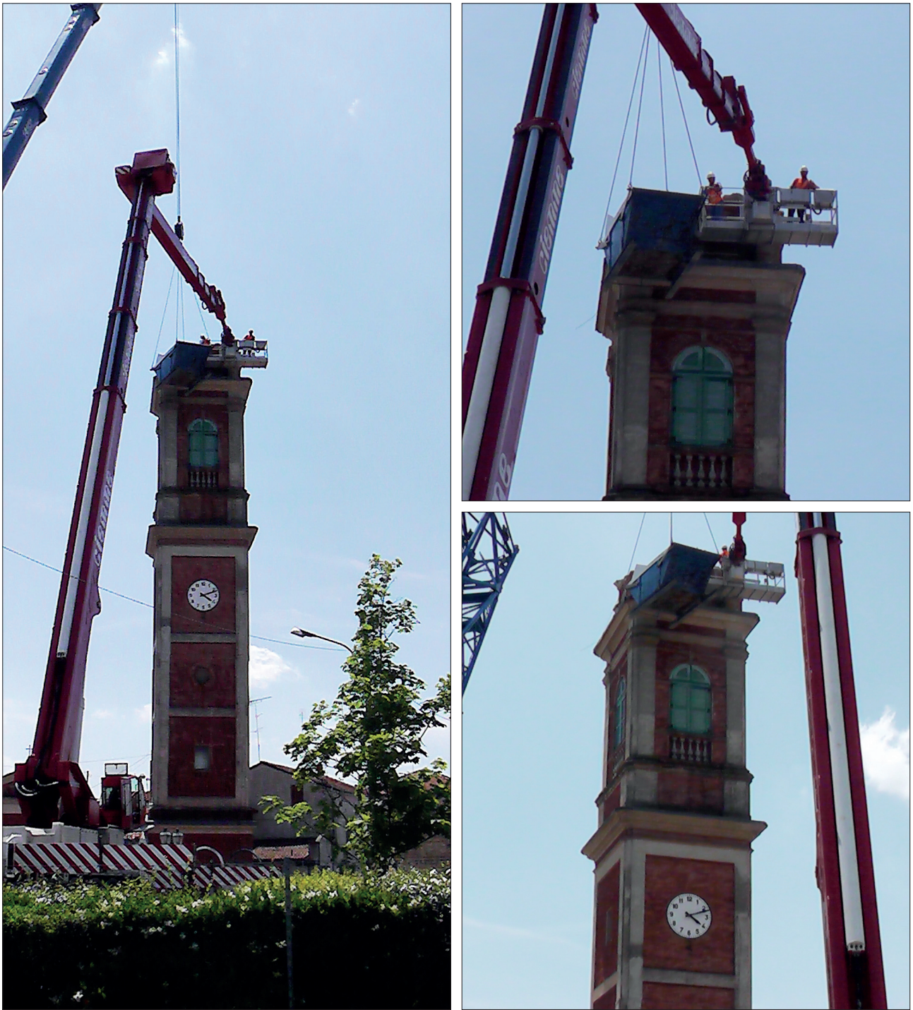
FIGURE 6 Controlled demolition in the San Martino di Tours church bell-tower in Buonacompra (Cento, Ferrara)
