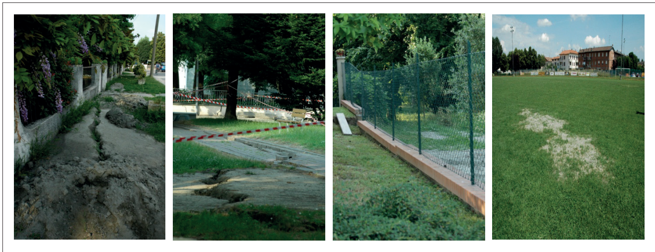
FIGURE 12 Sant'Agostino Municipality: cracks with sand spill that affected the buildings and the road surface, and the sports field of San Felice
