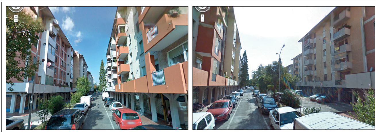
FIGURES 21-22 The CE.RES. residential complex in Cento
