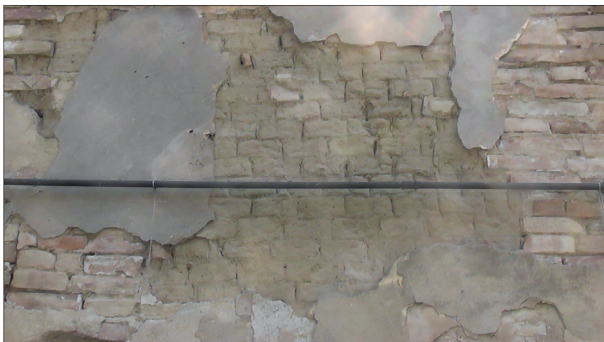
FIGURE 3 Adobe bricks observed in Casumaro (Cento)
