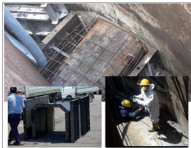
FIGURE 10 Crossing channel of intermediate section in the existing flow splitter
