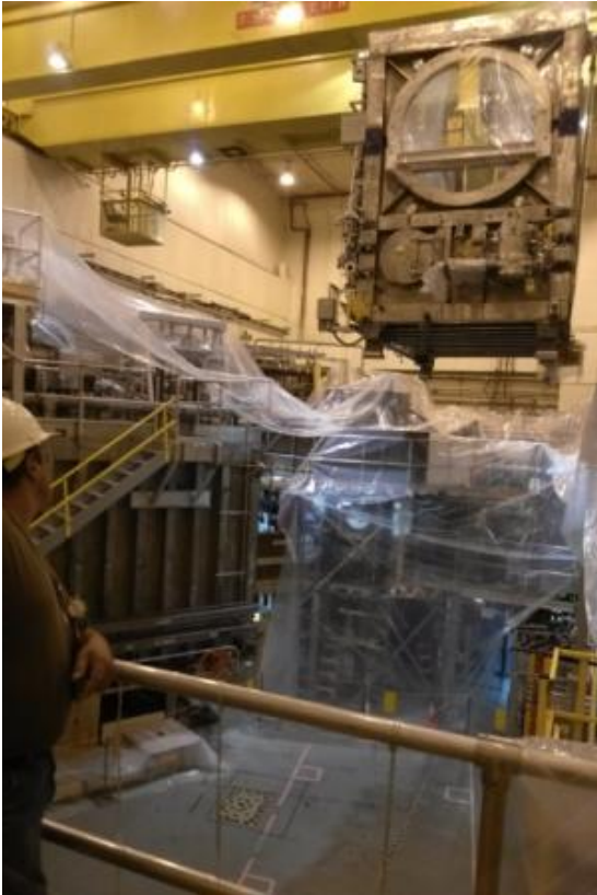
Beam Box being lifted over NSTX
