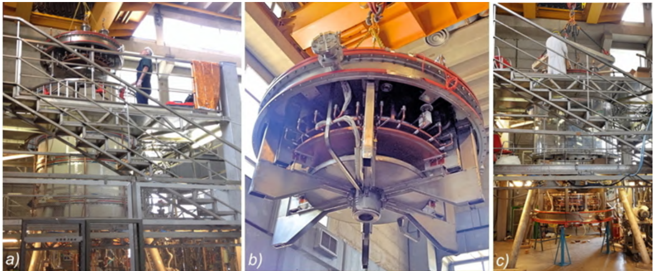
Figure 3. (a) The annular anode being lowered on the Aluminium vacuum vessel (May 2015). (b) Image of the copper anode, on the rear side of which white Teflon blocks and tubes insulate the gas-puffing system from the upper lid; the metal disc below is the PF3.1 coil and the cylinder the PF2 mirror coil, through whose hole the plasma emerges in the equatorial section of the machine. (c) The annular cathode, below the machine, being lifted into the vacuum vessel.
